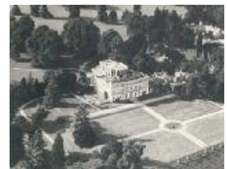
Gatton Hall, 1930 The hall was destroyed by fire in 1934.
