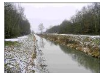
The catchwater drain Burton
